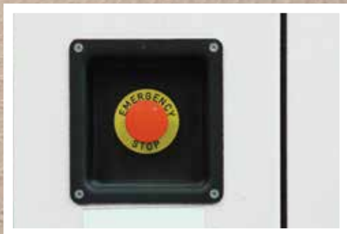
Emergency stop button placed on the outside of the control panel
