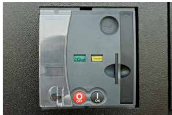
▲ Motorized circuit breaker for synchronization of generating sets
