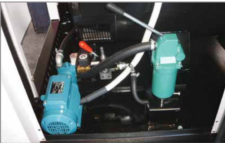
Automatic fuel refilling kit consisting of electric pump, manual pump, 4-level switch, electronic controller
