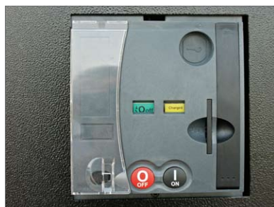
▲ Motorized circuit breaker for synchronization of generating sets
