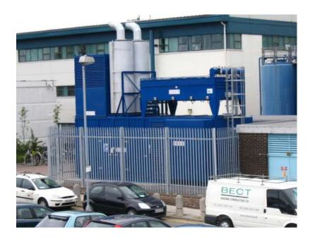
Power Back up for a major teaching hospital. Set is 3.14MVA in a 30ft custom built container with acoustic level 75dbA @ 1 metre.
